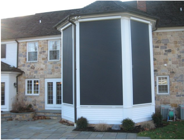
Screen fully lowered down
