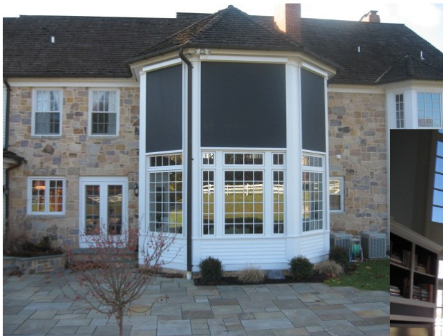
Screen partially lowered down
